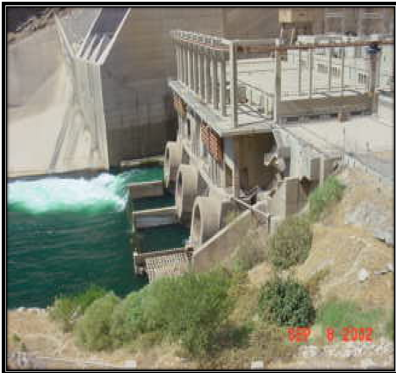
Derbendikhan Hydro Power Station
