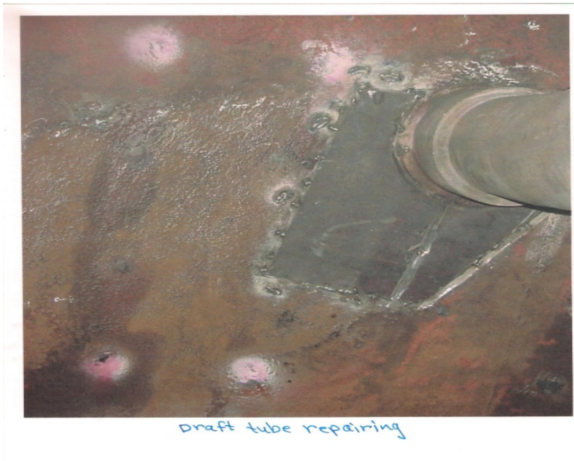
Draft tube repairing (plate 12)
